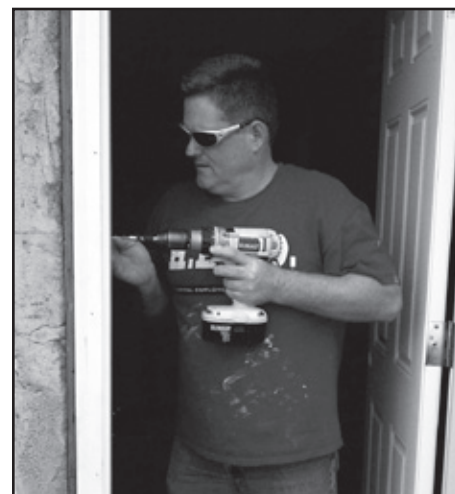
▶ Several new doors installed during Christmas in October will help Rosedale residents keep the cold out this winter.
